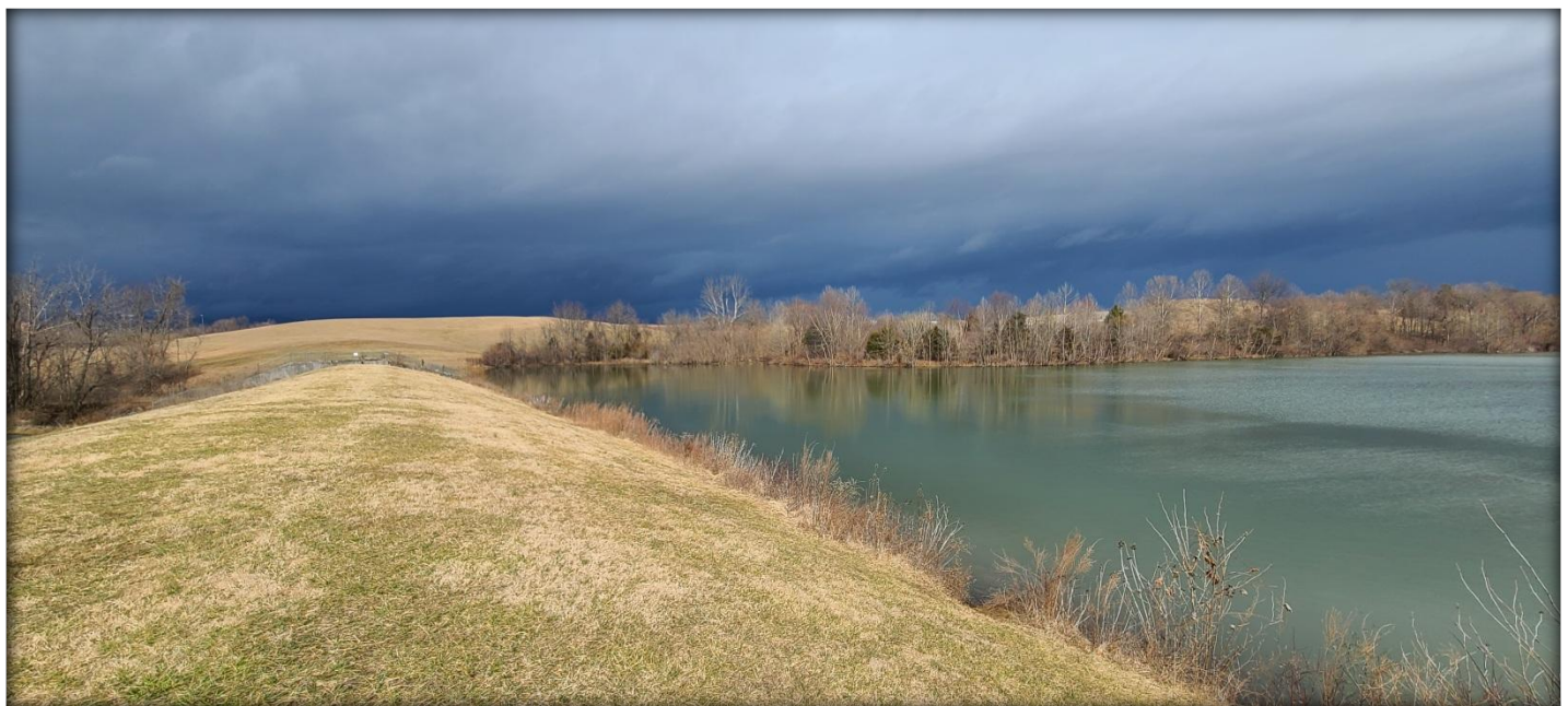
Greenfield Lake and dam, Botetourt County
